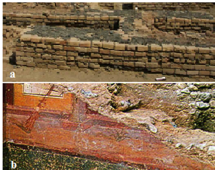
Figure 1. Three layered walls which improve the seismic behaviour, (a) Sumerian wall; (b) Roman wall
